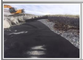
These works were designed to strengthen a portion of the existing Phase 2 works, carry out repairs to areas of the defences and prevent the continued erosion of beach material from the western boundary of Benbecula Airport on the Western Isles.
