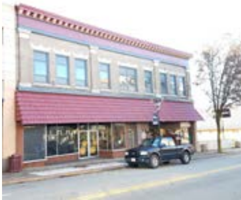
139 West Crawford Avenue New Windows, Accessible Doors
