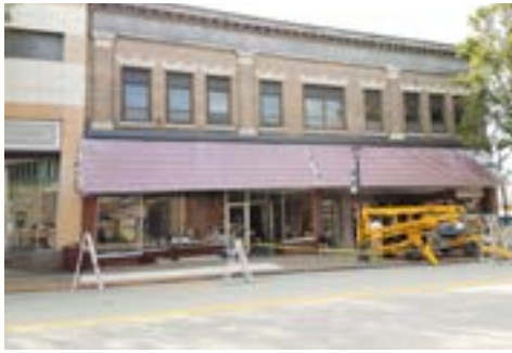
119 West Crawford Avenue Restored Cornice, Metal Awning
