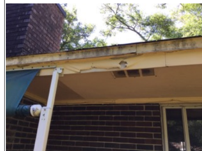
Fascia has wood rot on North West corner of roof
