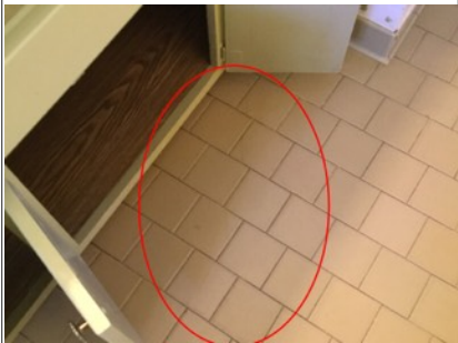
Cracked floor tile
