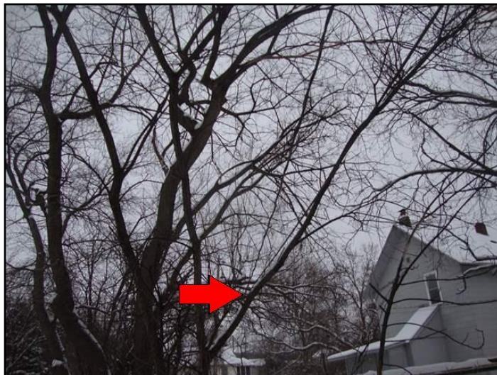
42. Branches, vines interfering with wires
