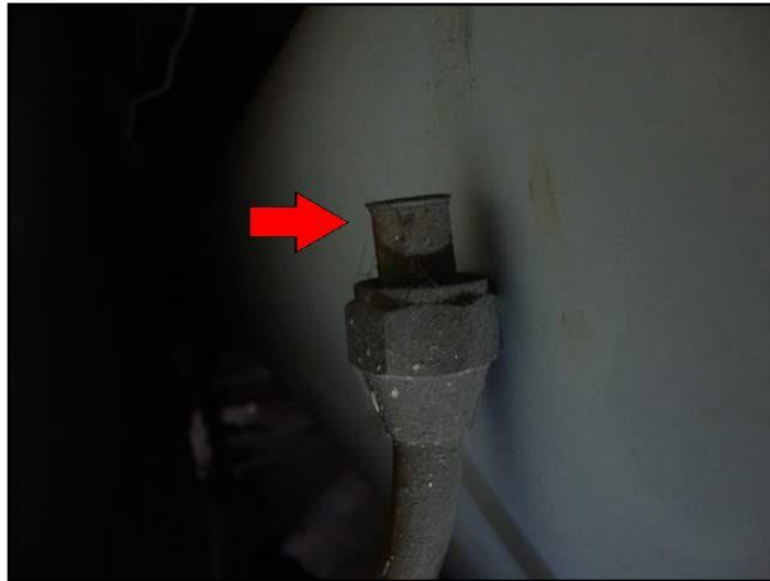
94. Improper connections
