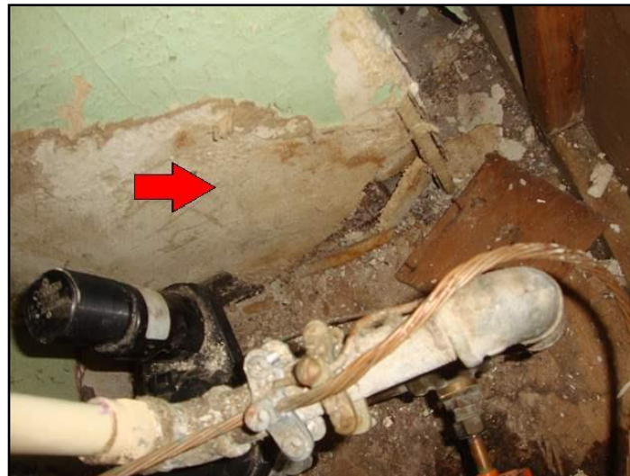
101. Water damage
