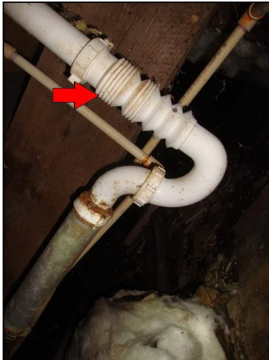
89. Nonstandard materials and patches
