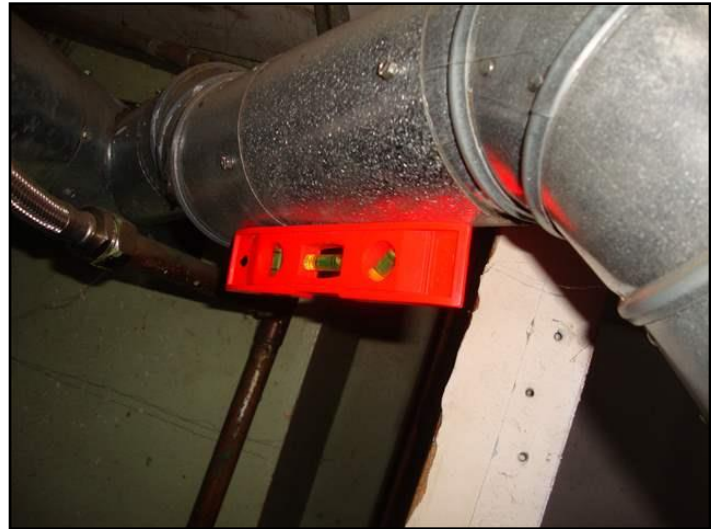
65. Poor slope
