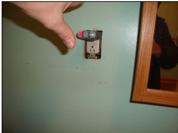
60. Ground Fault Circuit Interrupter (GFCI)...
