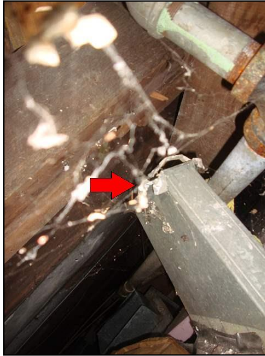
68. Disconnected ducts
