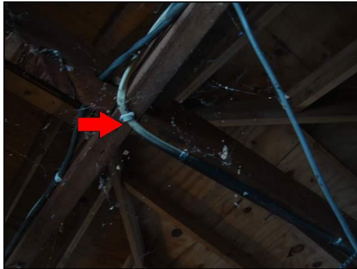
47. Exposed on walls or ceilings
