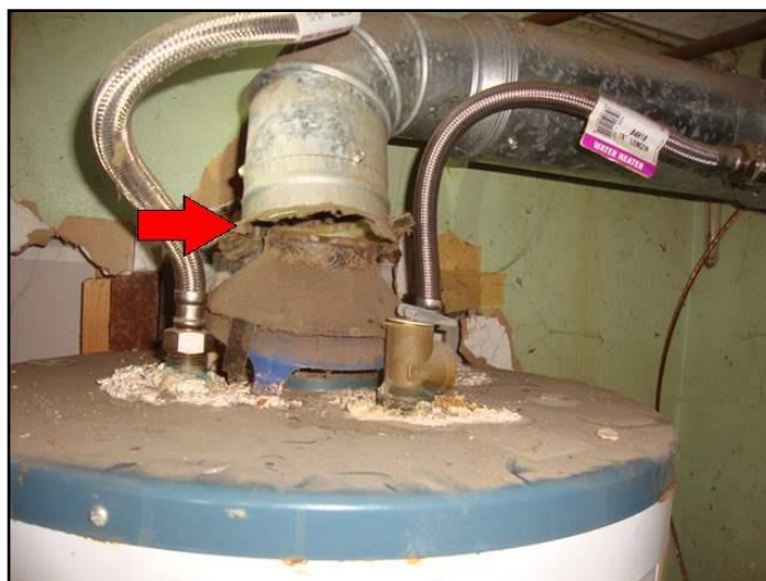
85. Poor connections
