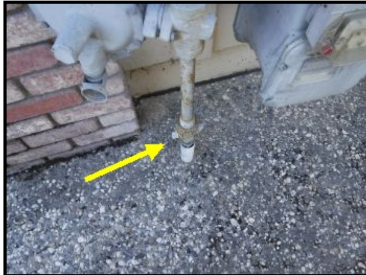
Main gas shut off. To turn of main gas shut off, turn valve so that flat area of the valve is perpendicular to the pipe. Make sure special wrench is always available in emergency.
