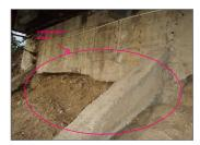
The steel plates on the top of the caissons are being deteriorated by rust, and should be serviced and monitored. This is important, because rust is progressive and could lead to a catastrophic structural failure.
