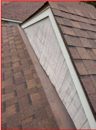
The wood siding on the garage is in poor shape.
