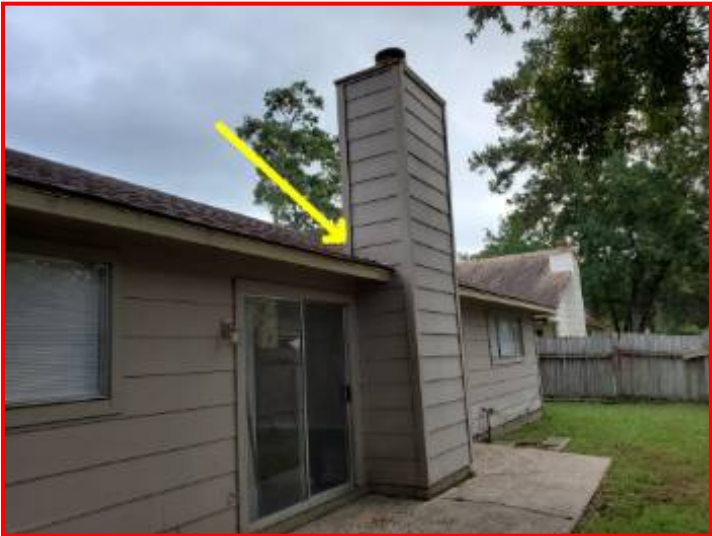
Siding is damaged at chimney.
