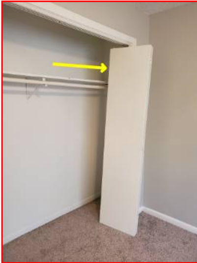
Closet door is off the hinge in front bedroom.
