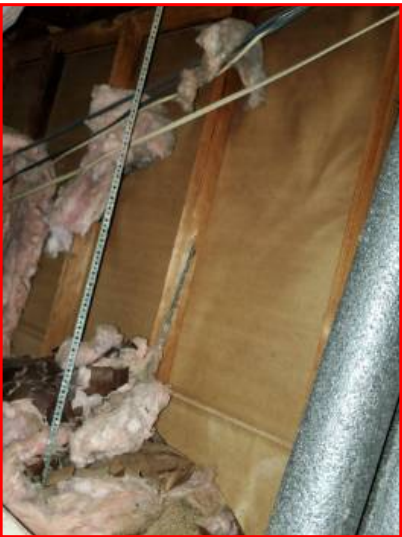
Insulation has fallen down.
