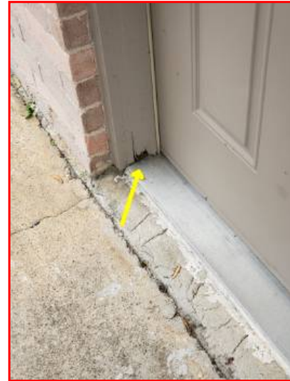
Trim around kitchen walk door needs replaced.
