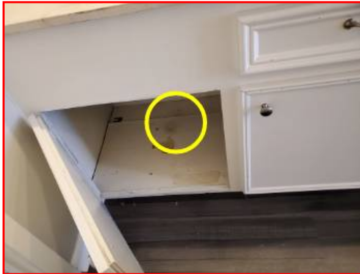
Drain leaking under master bathroom sink.
