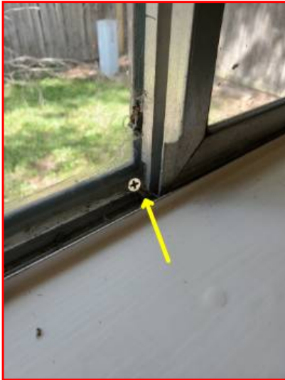
One or more windows had a screw stop installed.
