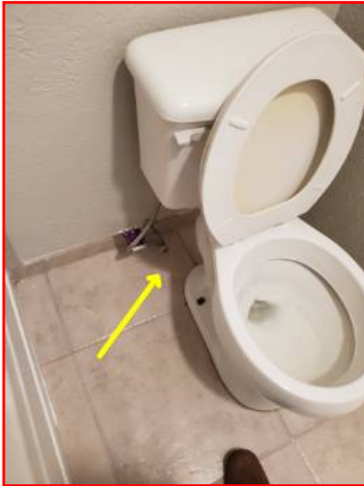
Toilet leaks on to the floor when flushed
