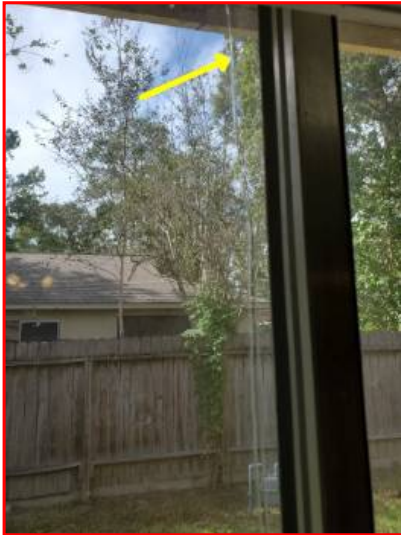
Cracked and/or broken glass was observed on one or more windows. Master bedroom.
