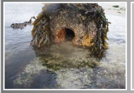
Installation of replacement outfall pipe. The works were required to work with the tide timetable . With limited shift times available to pour concrete. A section of the outfall was removed via hydraulic breaker and replaced with new shutter and concreted.
