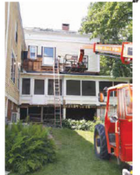
Exterior photo of restoration work in progress.
