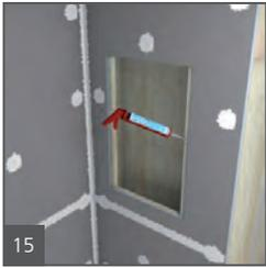
wedi Niches are installed in a cut out in the wedi wall and attached with it's flange right into the center of 16 o.c. studs. wedi Joint Sealant is set along the connection of wall to niche.
