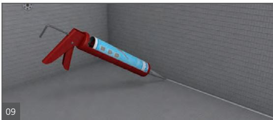
09 Apply continuous 1/2" beads of sealant between all connections of panels and install with tightly butted seams. Excess sealant must be spread flat with a putty knife. All seams and fastener heads in the assembly are covered with a secondary 1/2" bead of sealant and spread flat. The seams should be covered 3/4" to 1" on either side of seam. All fastener/washers are covered with sealant stretching 1" over the washer edges.
