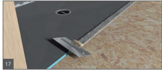
Apply thinset mortar over wood subfloor and reaching 4" into the wedi Fundo Ligno shower base. Fill the wedi Fundo Ligno channel with thinset or a strip of sealed on wedi Building Panel and apply thinset mortar to the lower corner of the wedi wall panels left and right of any entrance using 1/4" x 1/4" notch trowel.
