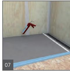
Set up a continuous 1/2" (13 mm) bead of wedi Joint Sealant at the perimeter channel and only in areas where you can immediately install a wedi Building Panel into the fresh sealant.
