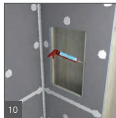
wedi Niches are installed in a cut out in the wedi wall and attached with it's flange right into the center of 16 o.c. (406 mm) studs. wedi Joint Sealant is set along the connection of wall to niche.
