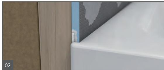
Measure and cut wedi Building Panel to fit the 16 inch o.c. framework (wood or metal). Notch out all panels if installed around the perimeter of a flange tub to integrate the flange and achieve a plumb wall with square and tight corners.
