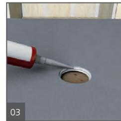
Set up a continuous 1/4" bead of wedi sealant along the top side of the wedi Fondos' valve groove profile.
