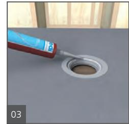
Set up a continuous 1/4" bead of wedi Joint Sealant along the top side of the wedi Fundos' valve groove profile.
