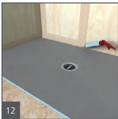
Set up a continuous 1/2" bead of wedi Joint Sealant along the pans channel on the outer perimeter and only in areas where you can immediately install a building panel into the fresh sealant.
