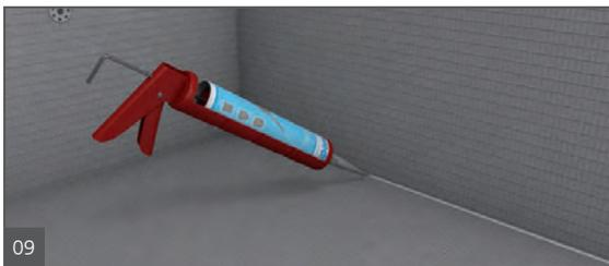
Apply continuous 1/2" (13 mm) bead of sealant between all connections of panels and install with tightly butted seams. Excess sealant must be spread flat with a putty knife. All seams and fastener heads in the assembly are covered with a secondary 1/2" (13 mm) bead of sealant and spread flat. The seams should be covered 3/4" to 1" (19 mm to 25 mm) on either side of seam. All fastener/washers are covered with sealant stretching 1" (25 mm) over the washer edges.
