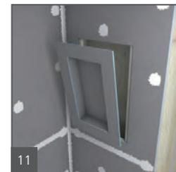
2 Fasteners each side of the niche are set to create a flush transition to the wall panels. Another 1/2" (13 mm) bead of wedi sealant is spread over fasteners and seams.
