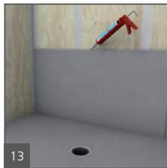
Push the wedi panel all the way into the channel of the shower base channel and its bead of sealant. Smooth out any pushed out sealant on inside seam using a putty knife. Fasten the panels directly to the studs starting 1 ft above the base and at a rate of 1 fastener per 1ft. One extra fastener is set into the seam to the next panel to crate a flush transition.
