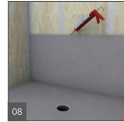
08 Push the wedi panel all the way into the channel of the shower base channel and its bead of sealant. Smooth out any pushed out sealant on inside seam using a putty knife. Fasten the panels directly to the studs starting 1 ft above the base and at a rate of 1 fastener per 1ft. One extra fastener is set into the seam to the next panel to create a flush transition.
