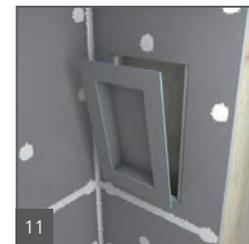
11 2 Fasteners each side of the niche are set to create a flush transition to the wall panels. Another 1/2" bead of wedi sealant is spread over fasteners and seams.
