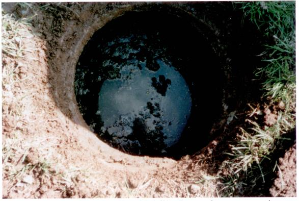
2) The tank was reopened 25 days later. Most of the build-up is gone and you can now see a large percentage of water. Since some solids remained the tank was again treated with Bio-Clean.
