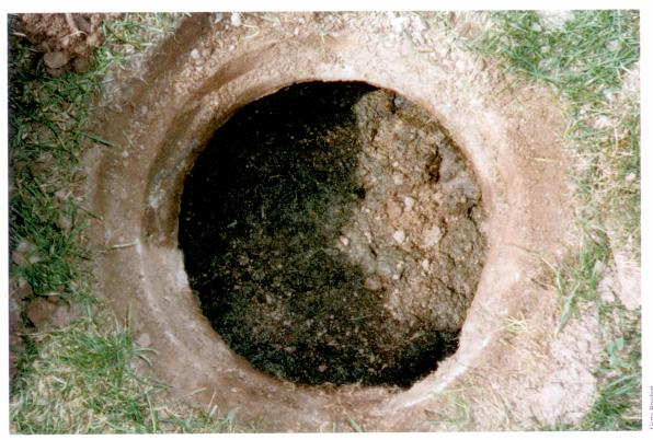
1) The inspection cover to a 1000 gal. septic tank was opened on Aug. 29th, 1995. As you can see there was a build-up of scum on the top of the tank. Using a spade it was discovered that the 'blanket' was hard and 10" - 12" (25-30 cm) thick! The scum blanket was broken up and treated with Bio-Clean, the revolutionary product for drains and septics.
