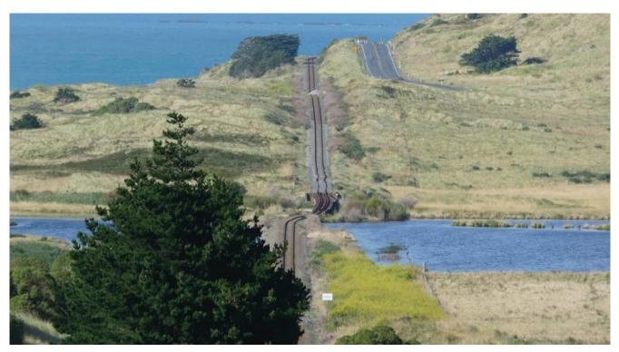
Bridge 129, Main North Line, moved approximately 0.6m horizontally and 2m vertically by the Kekerengu Fault during the November earthquake.
