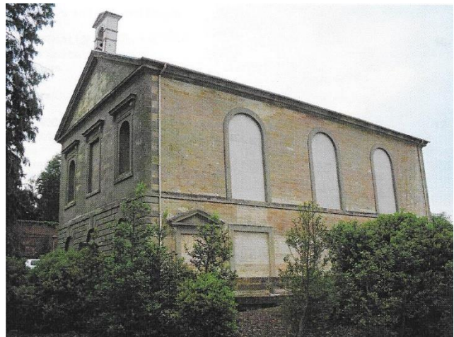
Figure 2 - Exterior of Chapel with windows boarded up
