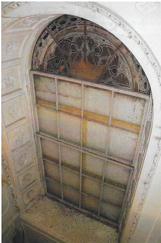
Figure 2 - Interior of window with original stained glass window
