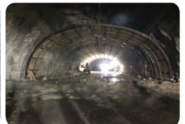
Drummanard Tunnel, KY
