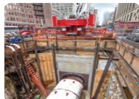
30th Street Rock Tunnel, NYC
