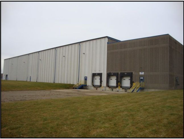
7 : Elevations - Typical Dock Bays
