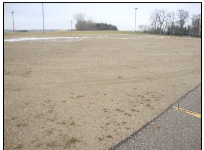
30 : Parking - Typical Gravel Paved Surfaces
