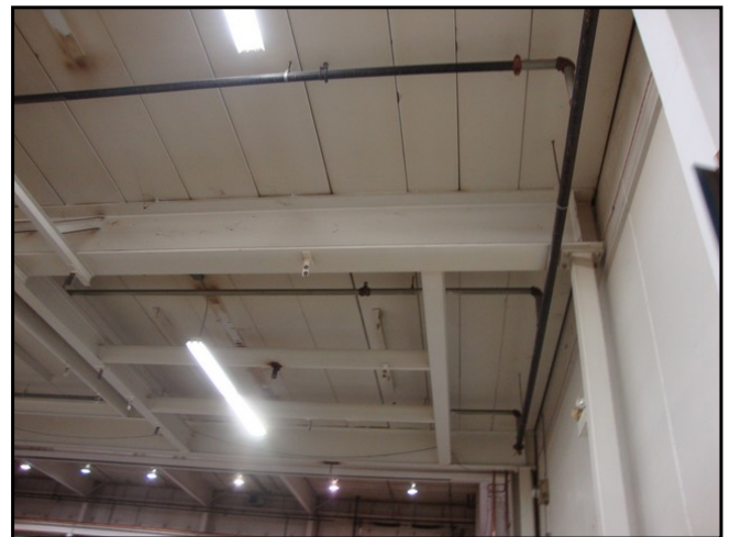
90 : Structure - Typical Warehouse Roof Framing
