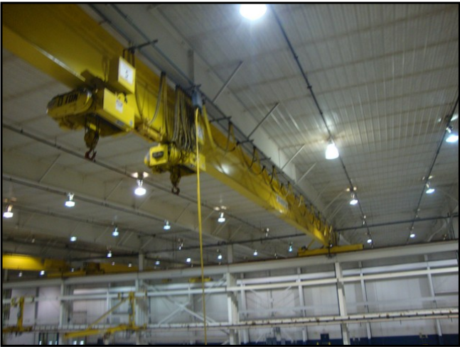
169 : Interior Photos - Typical Crane 1
