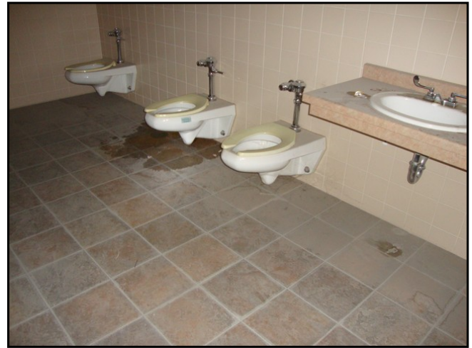
176 : Interior Photos - Unfinished 2nd Floor Restroom
