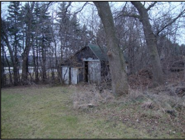
97 : Exterior - Abandoned Shed
