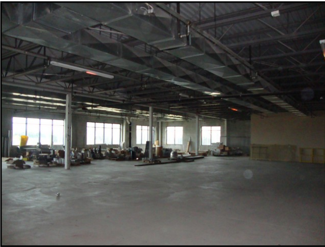
175 : Interior Photos - Unfinished 2nd Floor Office
