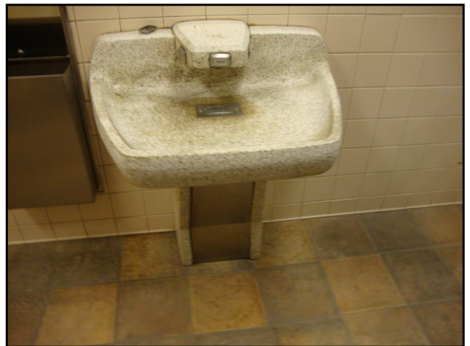
174 : Interior Photos - Typical Restroom 4
