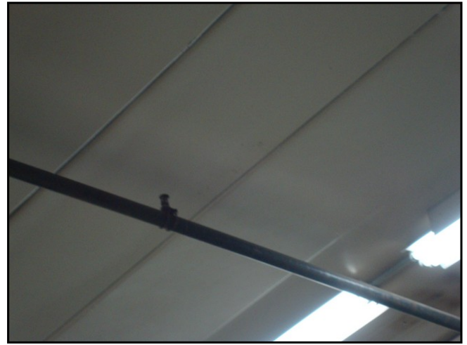
86 : Structure - Typical Floor Framing
