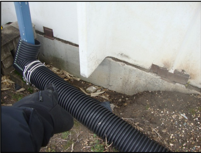
67 : Site - Storm Water Collection System 1
