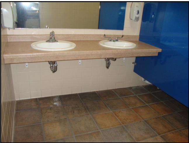
171 : Interior Photos - Typical Restroom 1
