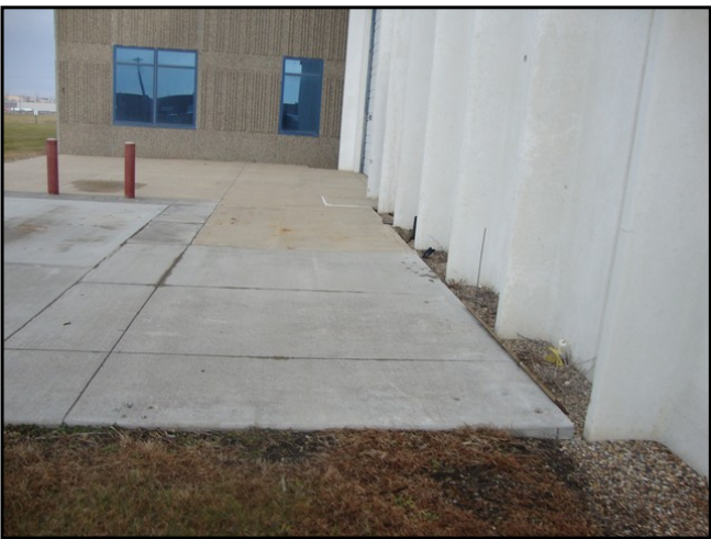
125 : Flatwork - New Sections
