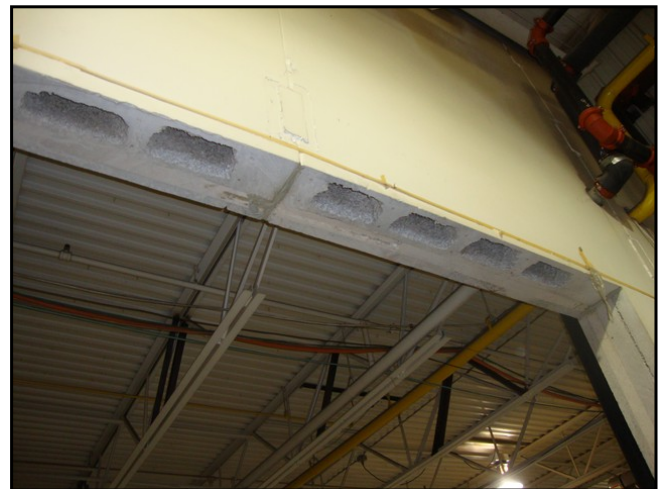
84 : Structure - Modified Opening at Addition
