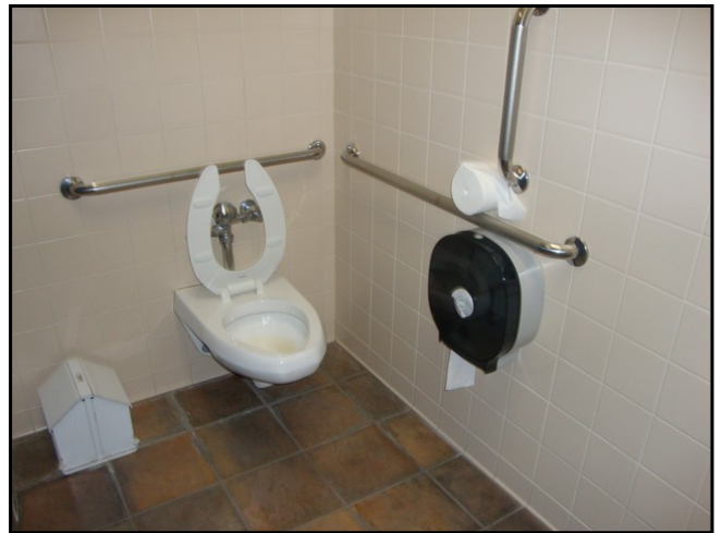
172 : Interior Photos - Typical Restroom 2
