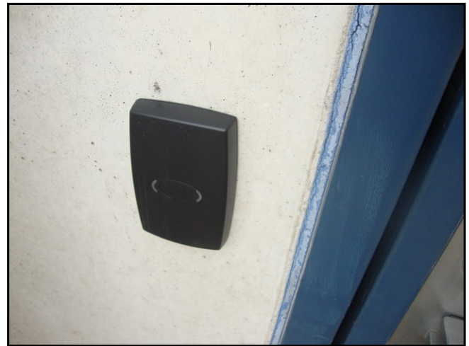
106 : Exterior - Secured Access
