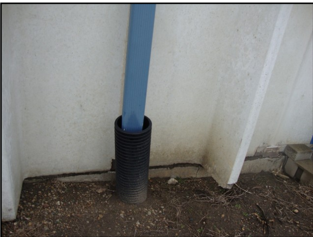
77 : Structure - Foundation Crack
