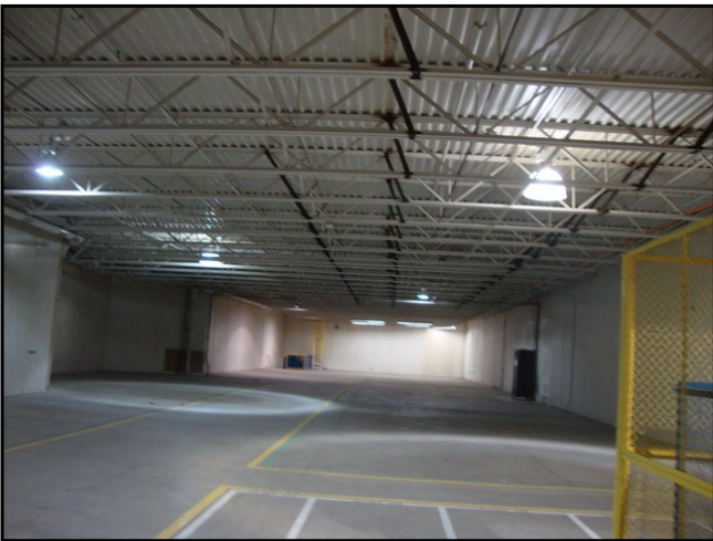
165 : Interior Photos - Mezzanine
