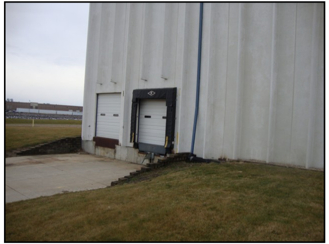
8 : Elevations - Southwest Dock Bays
