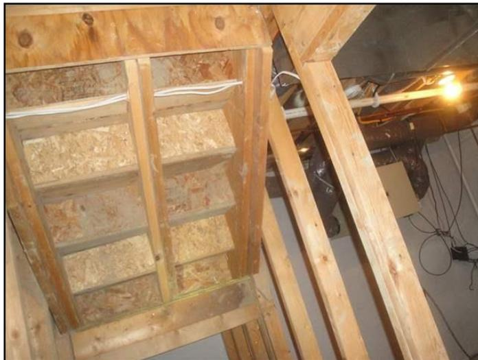
73. Drywall missing or incomplete on underside...
