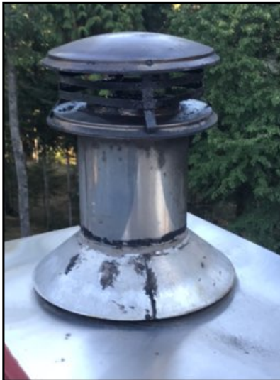
Melted and lot of cresote
