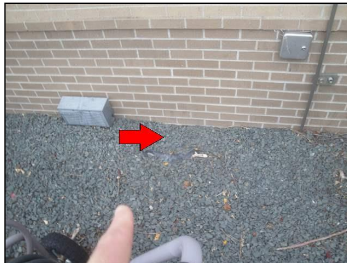
43. Improper grading
