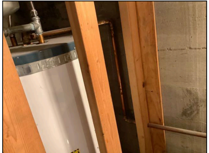
35. Discharge arrangement poor
