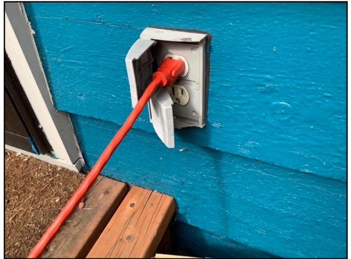
25. GFCI/GFI needed (Ground Fault Circuit...
