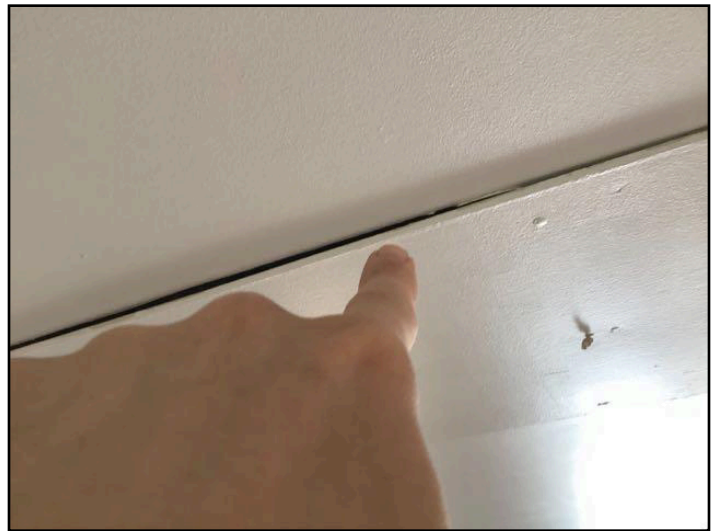
30. Inadequate insulation
