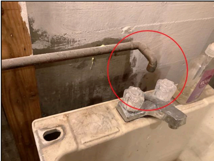
34. Discharge arrangement poor
