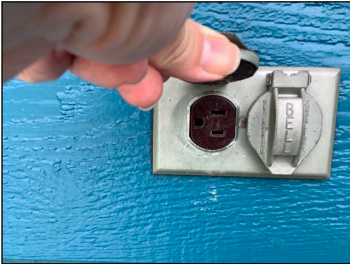
24. GFCI/GFI needed (Ground Fault Circuit...
