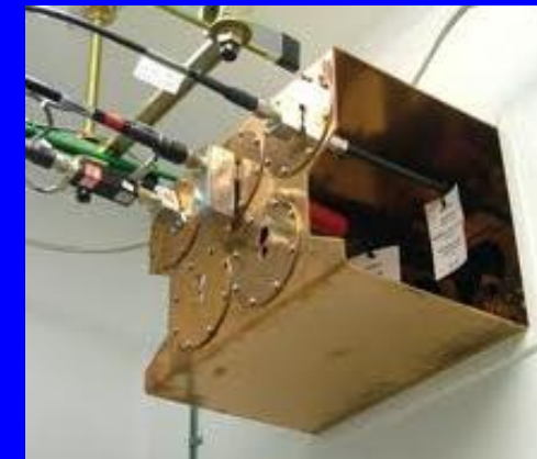
Typical copper-integrated Entry Panel Exterior View
