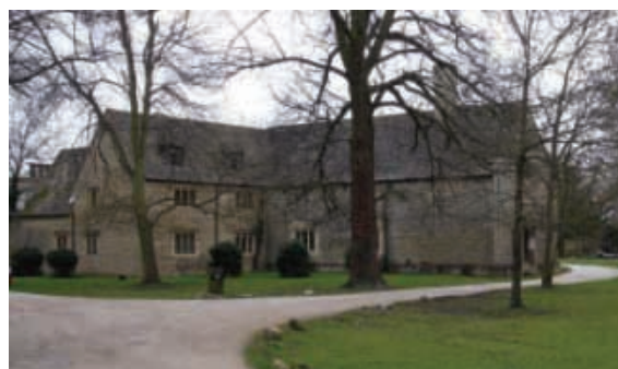
Outbuilding, now converted to residential properties, north of The Manor.
