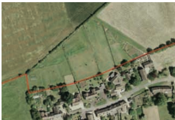
Aerial view of rear gardens of properties facing North Lane.
