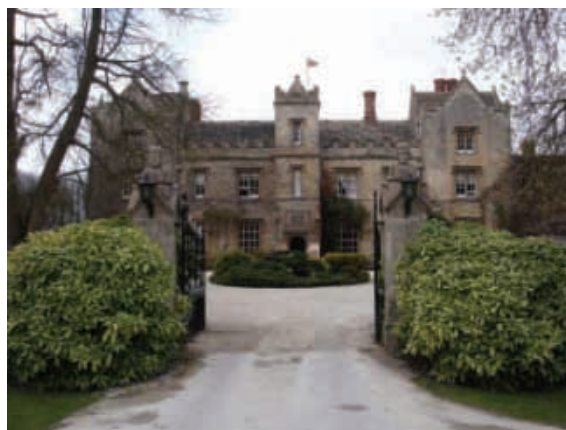
Weston Manor with Forecourt Wall.
