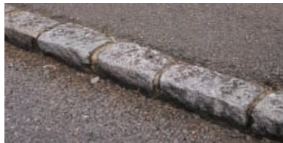
Granite setts define edge of footway.
