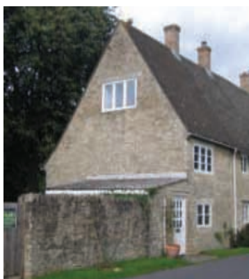
Existing steeply pitched roof of Mulberry Cottage.
