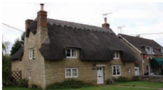
Willow Cottage with first floor eye brow dormers.
