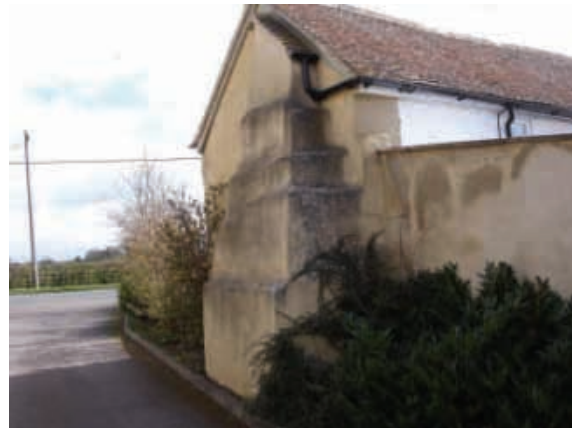
Tiered addition to the side of Mithian Cottage.
