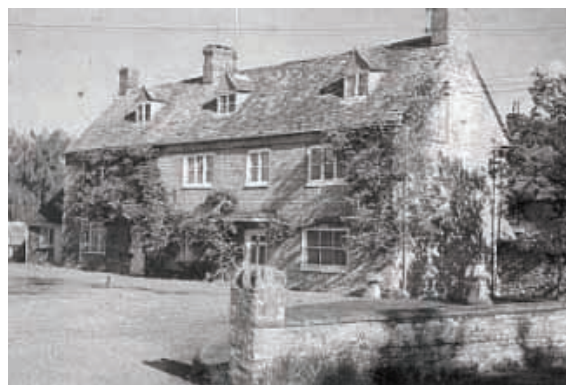
6 and 7 Oxford Court before its conversion
