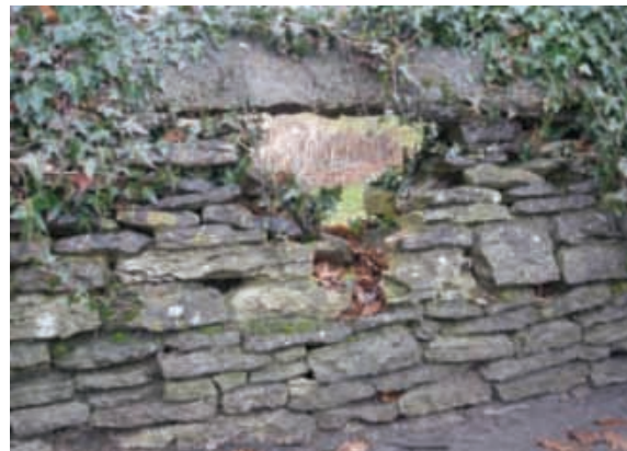
Failure of part of front boundary wall.
