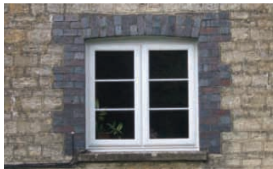
Vitrified brick detailing.
