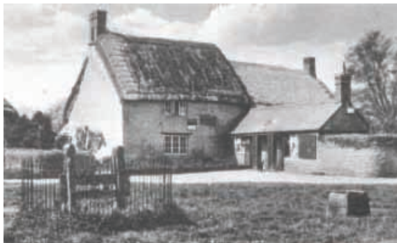
Historic photograph of Hazel Cottage. Taken from Weston Matters.
