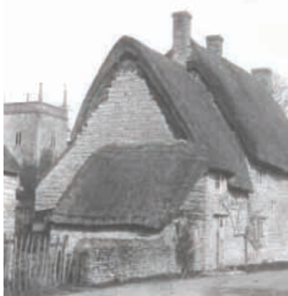
Original thatched roof of Mulberry Cottage.
