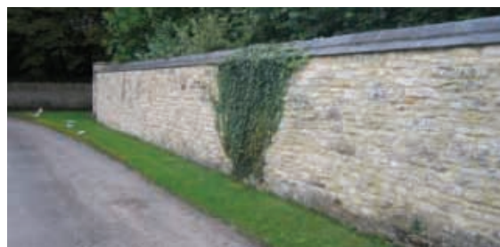
Boundary wall of the Vicarage with grey ridge tiles.
