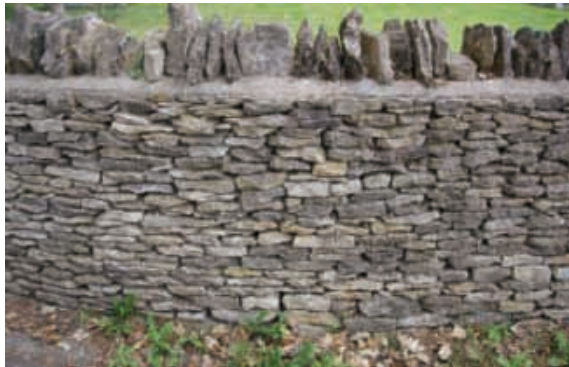
Stone laid on edge forms coping
