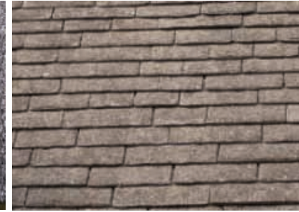
Newly laid replica slates.
