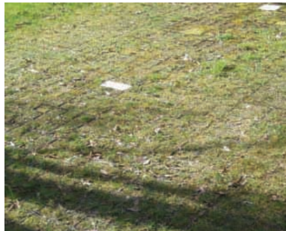
Grasscrete laid into verge to allow vehicular parking.
