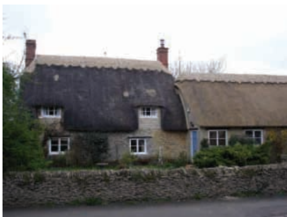
Rutland Cottage with newly thatched roof.
