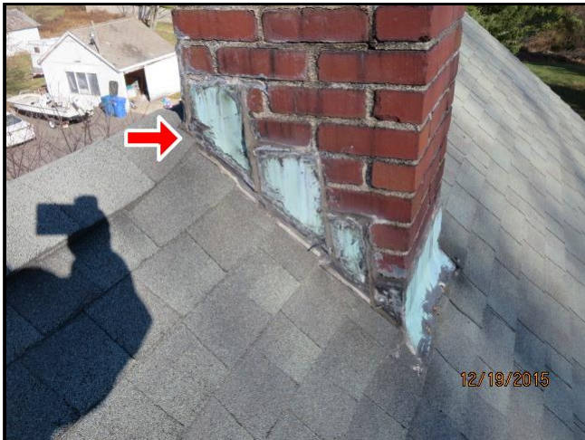
1.1 Item 3(Picture) Flashing
