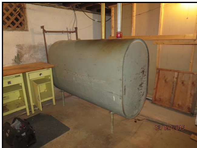
5.5 Item 1(Picture) Oil Barrel
