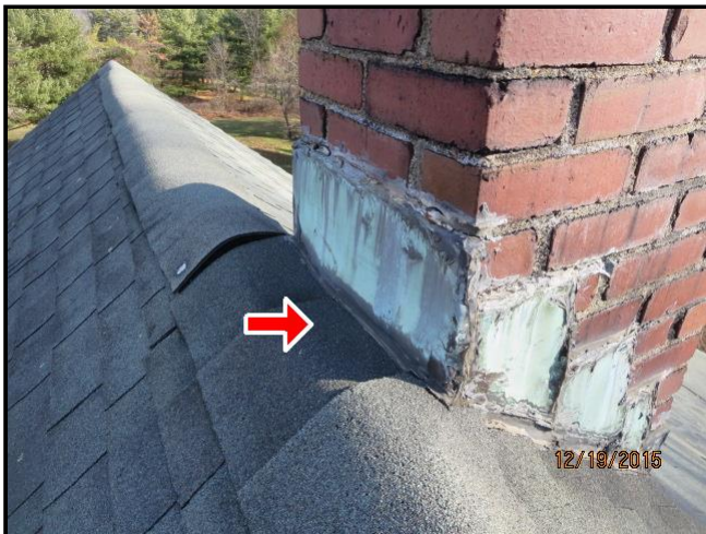
1.1 Item 1(Picture) Flashing
