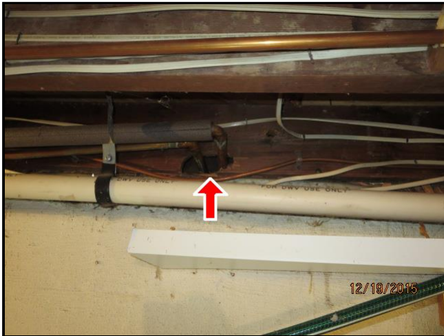
6.2 Item 1(Picture) Support Beam
