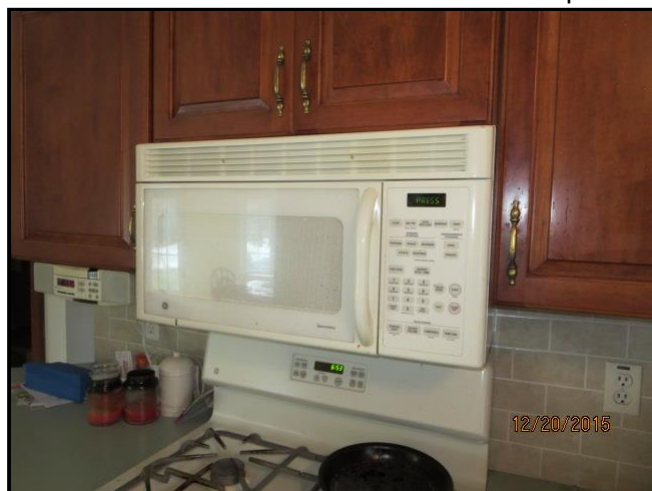
10.5 Item 1(Picture) Microwave
