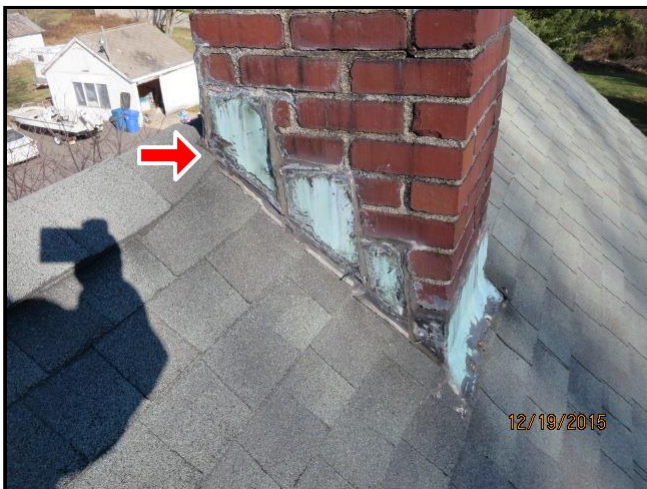
1.1 Item 3(Picture) Flashing
