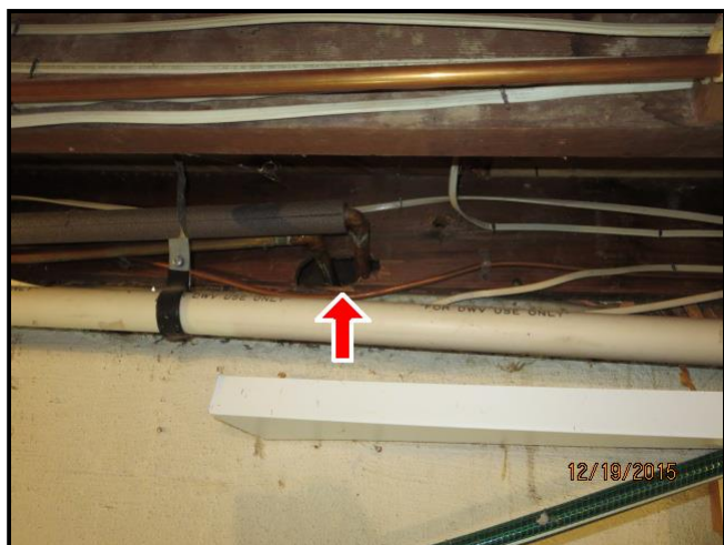
6.2 Item 1(Picture) Support Beam
