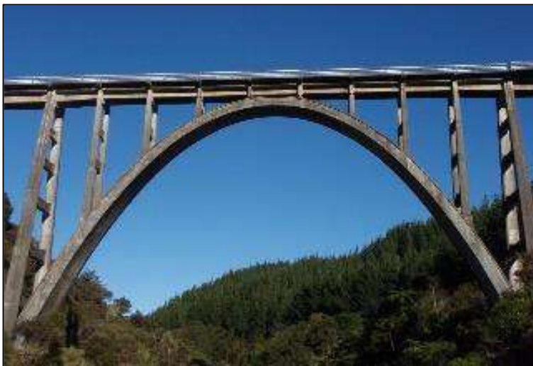
Photo 4.7 Bridge 264, the Kopuawhara Viaduct
