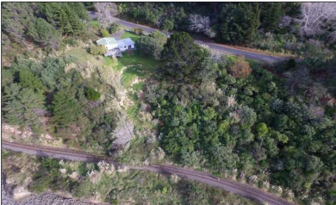
Photo 4.9 House site slump
