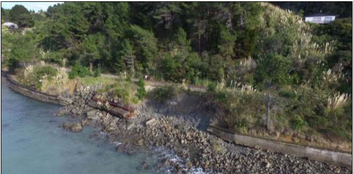
Photo 4.11 Erosion of the sea wall leaves the track exposed
