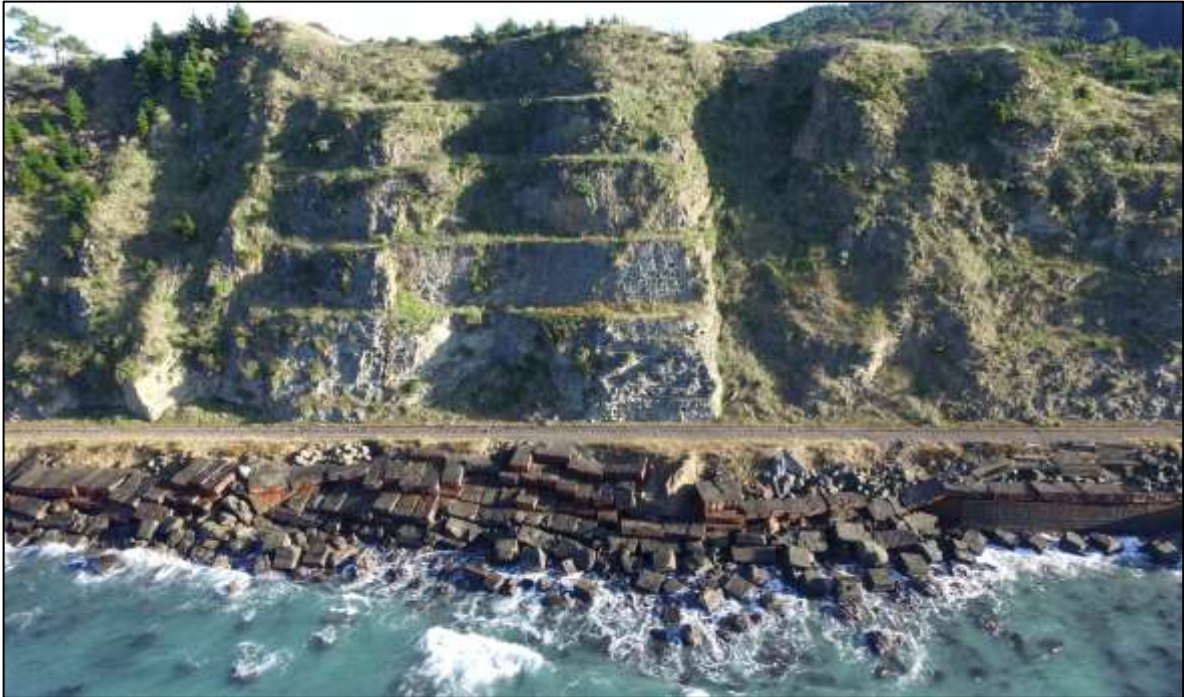
Photo 4.11 Erosion of the sea wall leaves the track exposed
