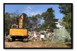
builders out there within the next week to plan the new building. Demolition should be finished by Thursday and the engineer with check the slab to see if it can be salvaged. If not, the building will be started from a new slab.
