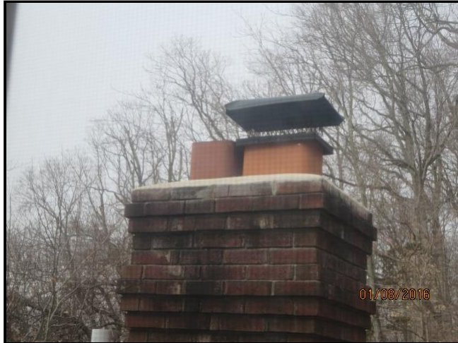
4.5 Item 1(Picture) Chimney
