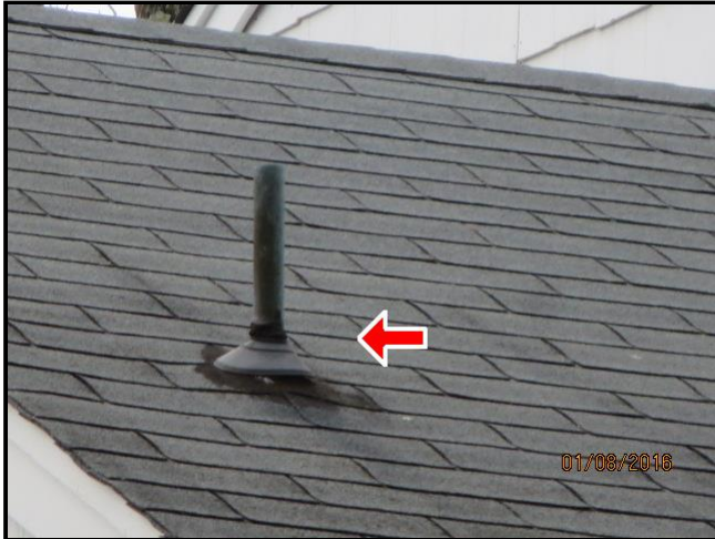
1.2 Item 1(Picture) Pipe Flashing
