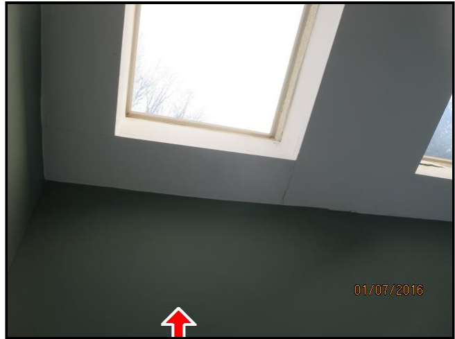
1.2 Item 4(Picture) Bath walls
