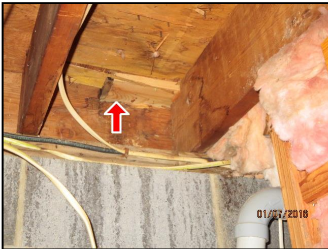
6.1 Item 6(Picture) Joist Repair
