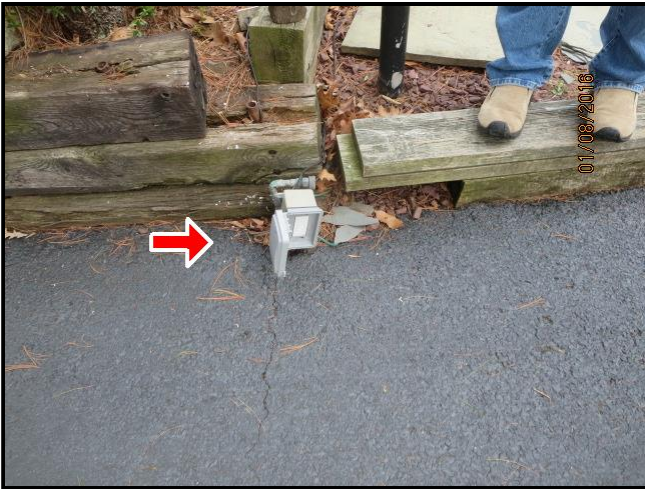
3.3 Item 7(Picture) Driveway outlet
