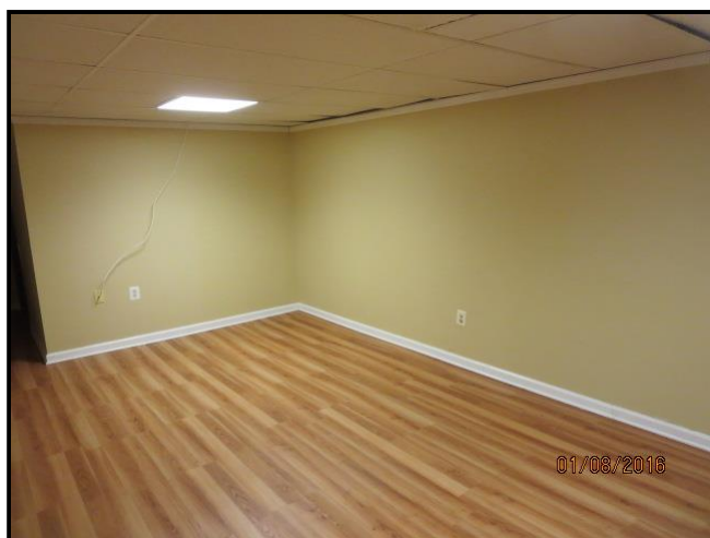
6.4 Item 1(Picture) Finished basement
