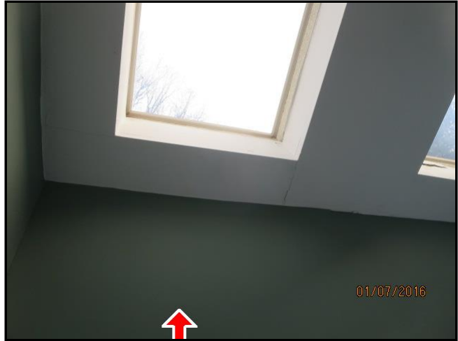
1.2 Item 4(Picture) Bath walls
