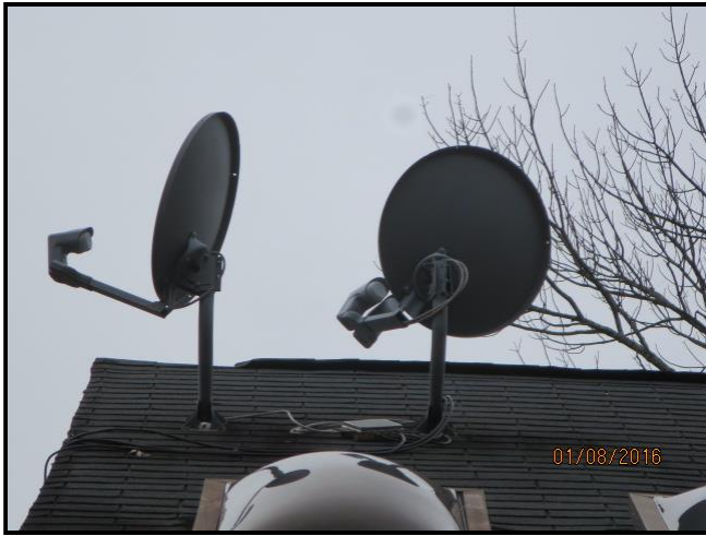
1.2 Item 2(Picture) Satellite dishes
