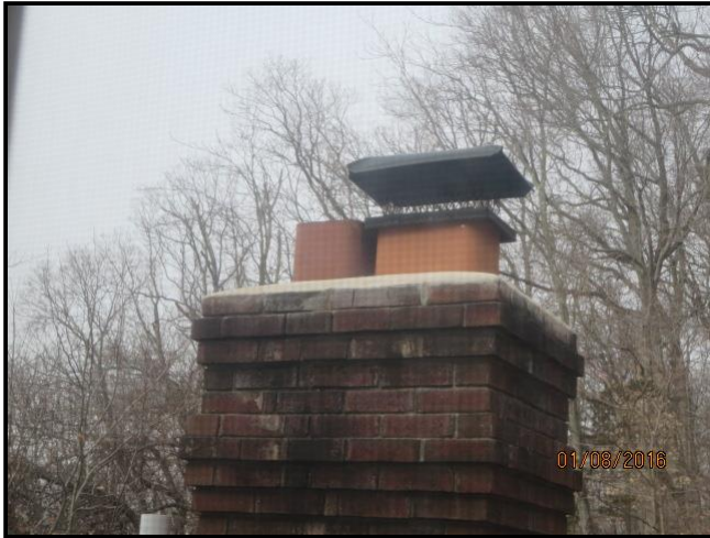
4.5 Item 1(Picture) Chimney
