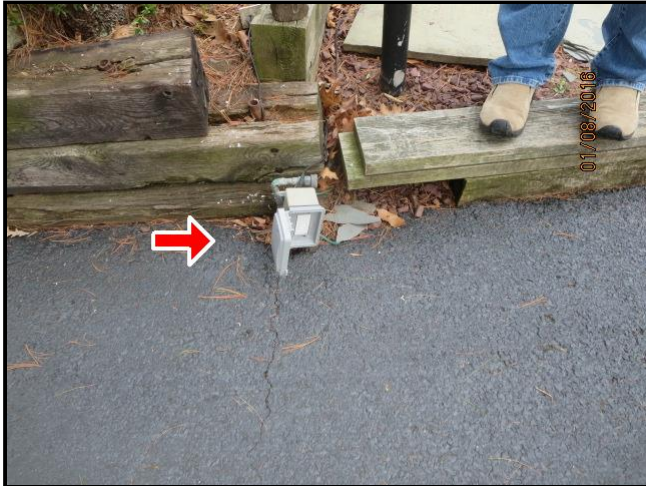
3.3 Item 7(Picture) Driveway outlet
