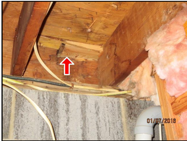
6.1 Item 6(Picture) Joist Repair
