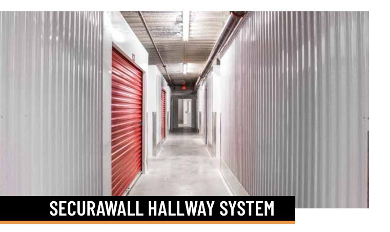
The Securawall System is a low cost, attractive divider partition for self-storage facilities. The panel is designed to lock together tightly at the side seams without the use of exposed fasteners, this hallway system ensures security without sacrificing function, quality, or aesthetics.
