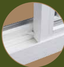
Ventilation limit lock closed
