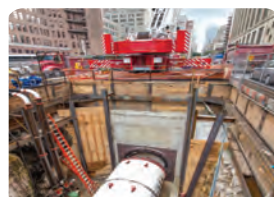
30th Street Rock Tunnel, NYC
