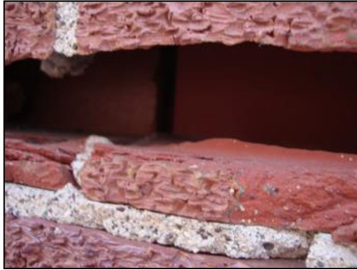
58. Water damage
