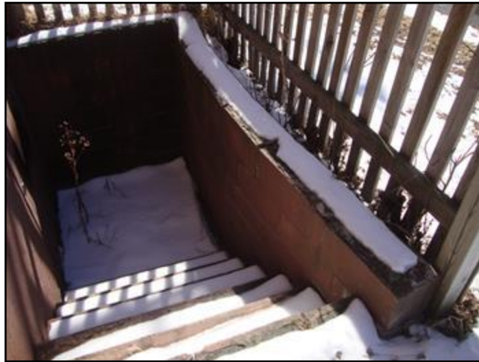
73. Missing drain
