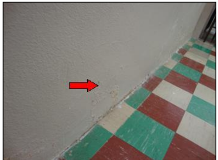
40. Efflorescence
