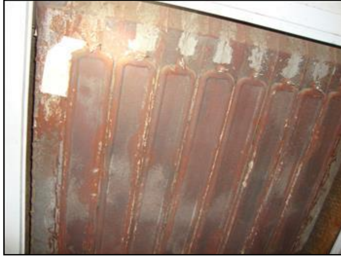
7. Corroded casing
