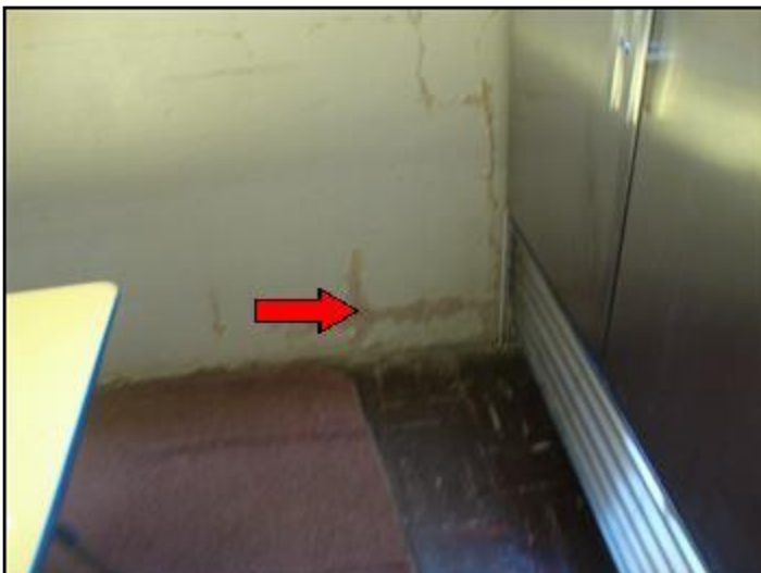
39. Efflorescence
