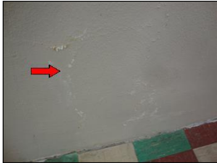
41. Efflorescence
