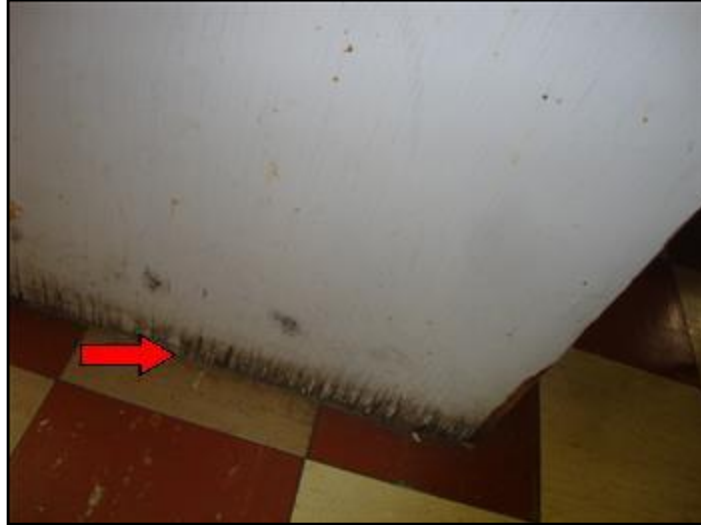
32. Water damage
