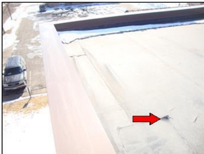
24. Open seams at lap joints
