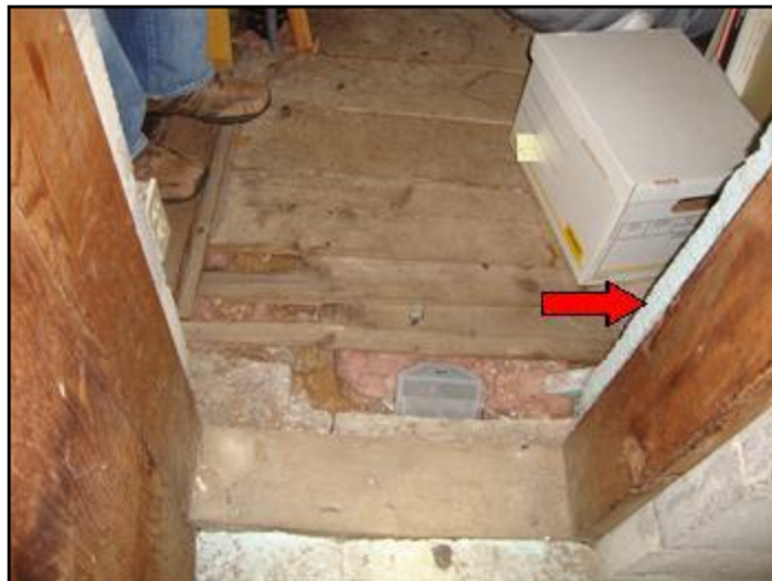
45. Exposed polystyrene foam insulation
