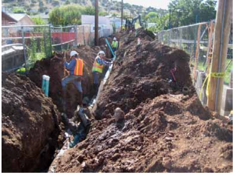
Crews at work installing a new wastewater collection line
