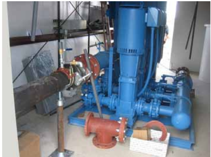
Bayard's 2009 improvements to the fresh water system: (Top) new fresh water booster building; (Bottom) fresh water booster pumps.
