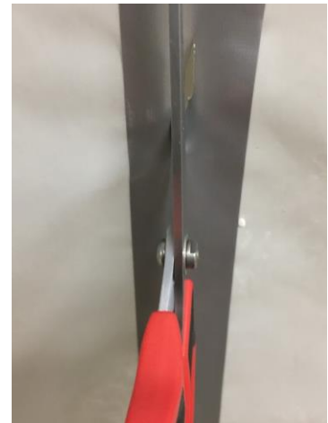
Step 19: cut an opening in the taped marking
