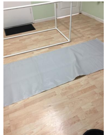
Roll 6 mil poly at least 36 inches past bottom
