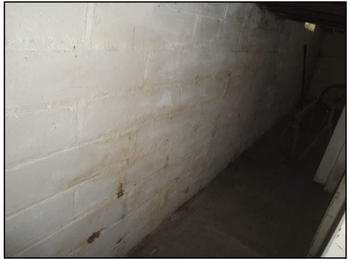
131. Efflorescence
