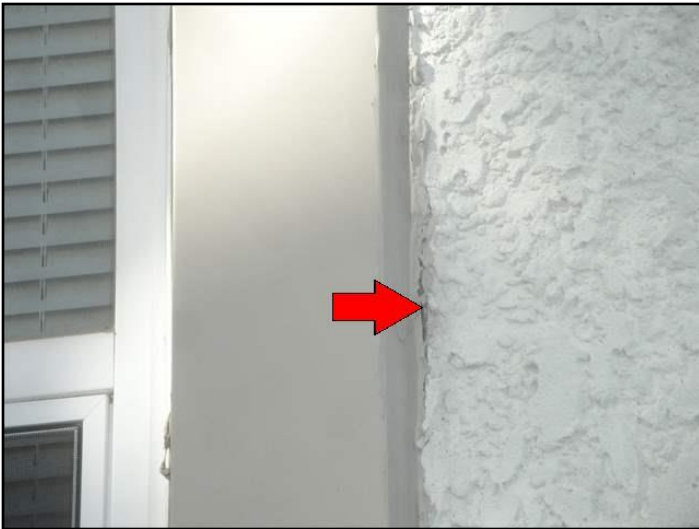
30. Caulking missing or ineffective
