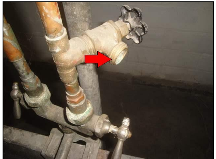
102. Backflow prevention missing
