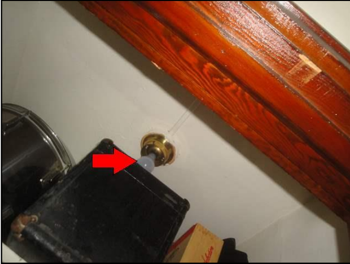
69. Improper closet lighting
