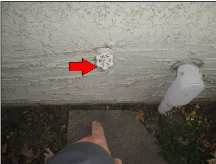
101. Backflow prevention missing
