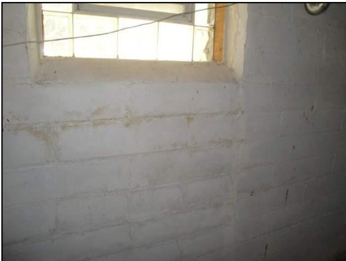
132. Efflorescence
