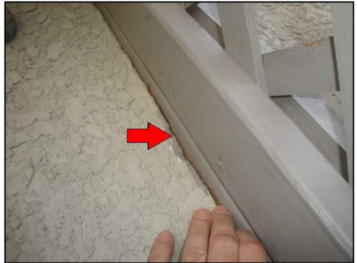
31. Caulking missing or ineffective
