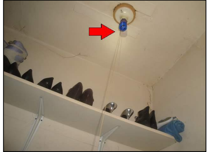
70. Improper closet lighting
