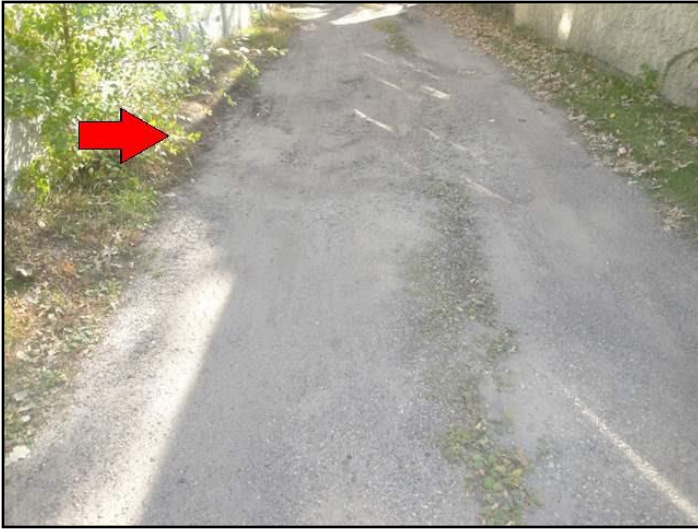
44. Improper slope
