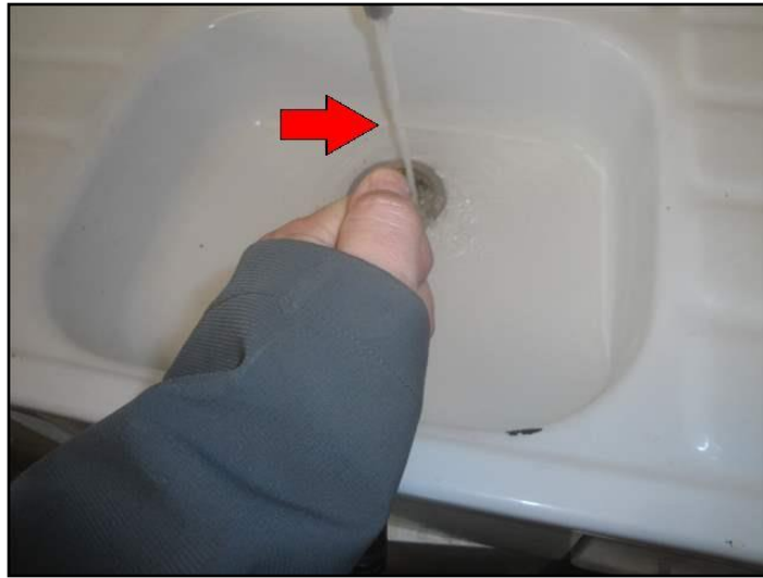
89. Poor pressure or flow
