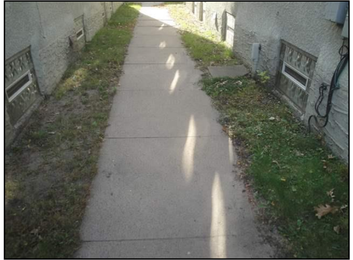
45. Improper slope
