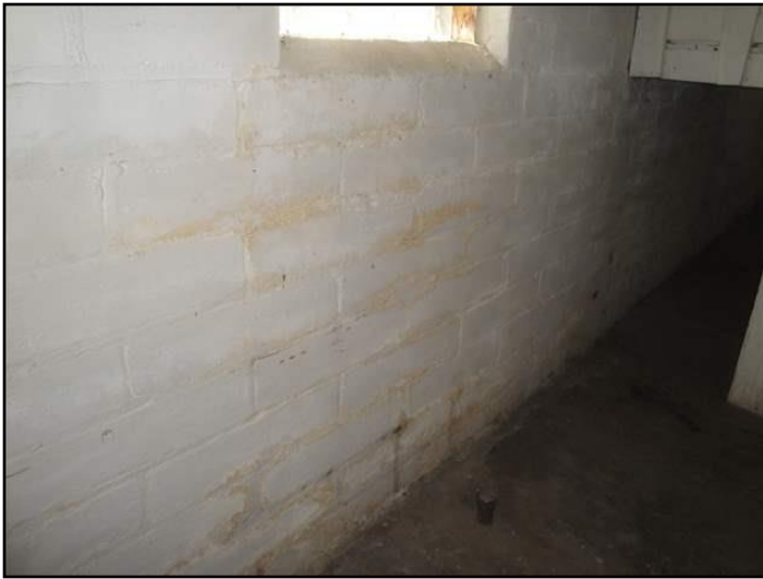
130. Efflorescence
