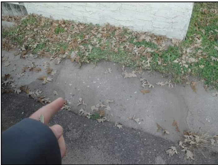
42. Improper slope
