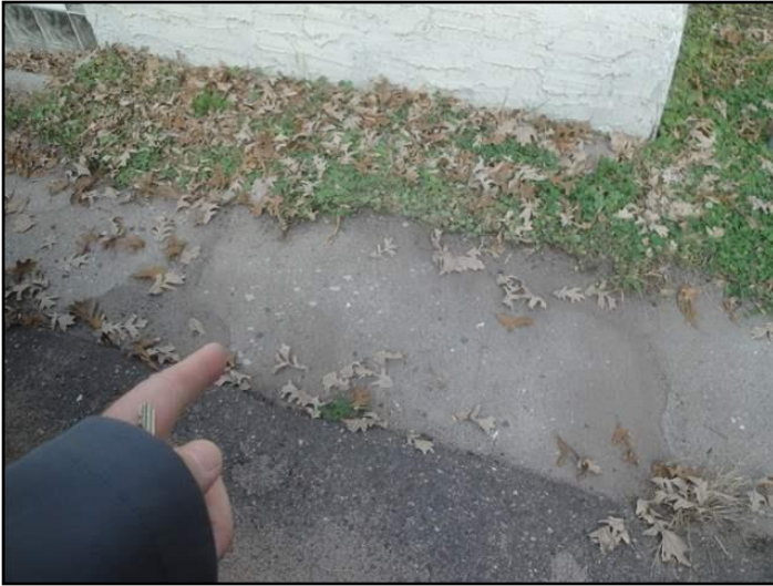
49. Improper slope or drainage
