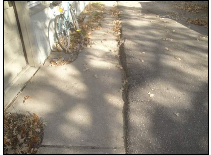
50. Improper slope or drainage
