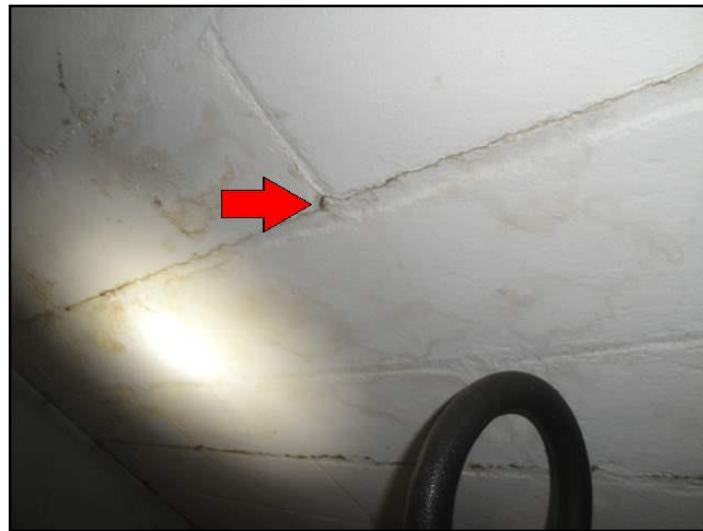
62. Cracked horizontally
