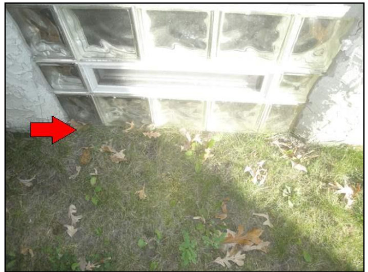
43. Improper slope
