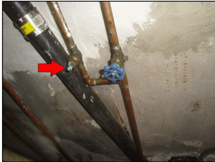
88. Damaged handle
