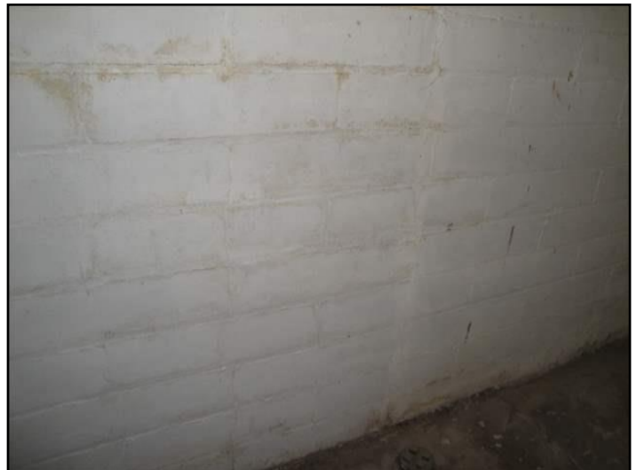
133. Efflorescence
