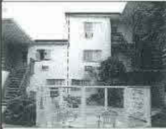
East Courtyard Wall East Stone Finish Panels Formed Cast In-Place
