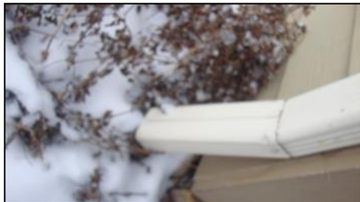
Downspouts end too close to building
