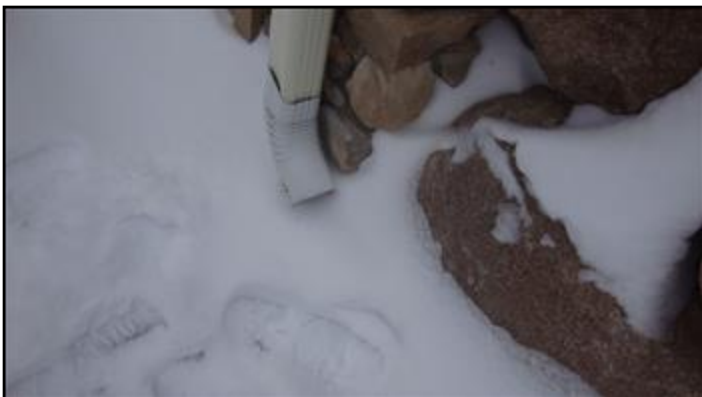
Downspouts end too close to building
