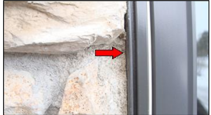
Missing, ineffective weep holes or flashings
