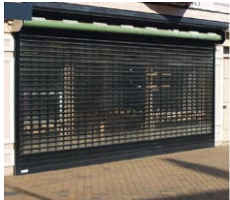
Photograph showing open grill which does not close the active frontage and provides security.
